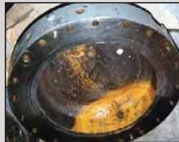
Corrosion caused by water in fuel
